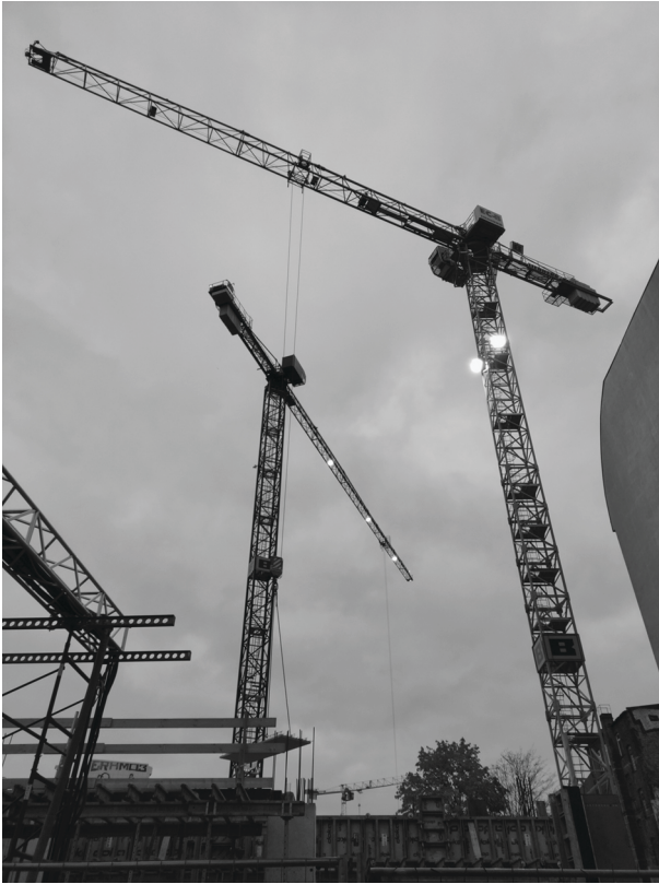
FIGURE 13.5 Vertical city. Construction site on Mariannenstraße at Skalitzer Straße (27 October 2021).
