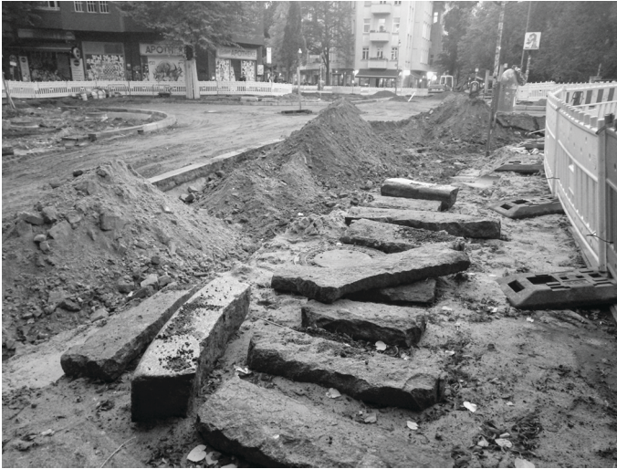
FIGURE 13.7 Demolishing old barriers. Construction site on Ohlauer Straße at Maybachufer (18 October 2020).
