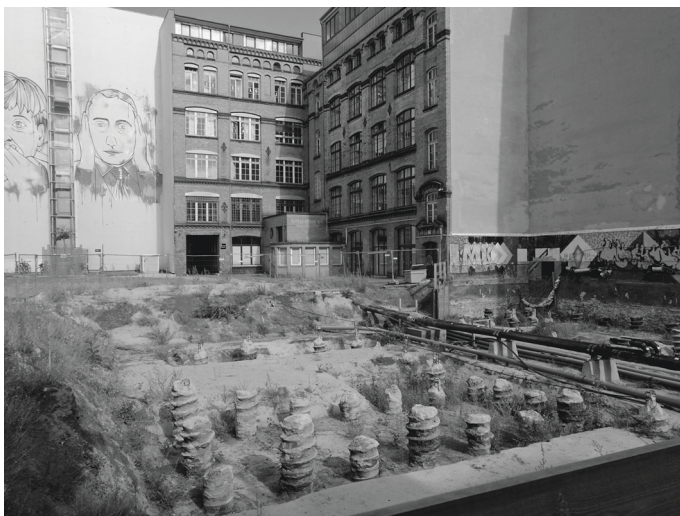
FIGURE 13.3 Processing soil I. Construction site on Adalbertstraße at Zentrum Kreuzberg (28 September 2020).
