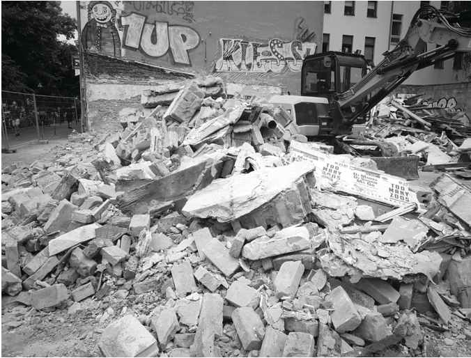
FIGURE 13.1 Pre-construction destruction. Construction site on Mariannenstraße at Reichenberger Straße (1 August 2019). For a full-color experience, please consult the digital version of the publication.
