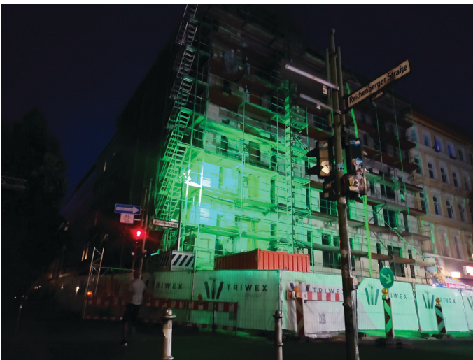
FIGURE 13.6 Monstrous surveillance. Construction site on Mariannenstraße at Reichenberger Straße (16 June 2022).
